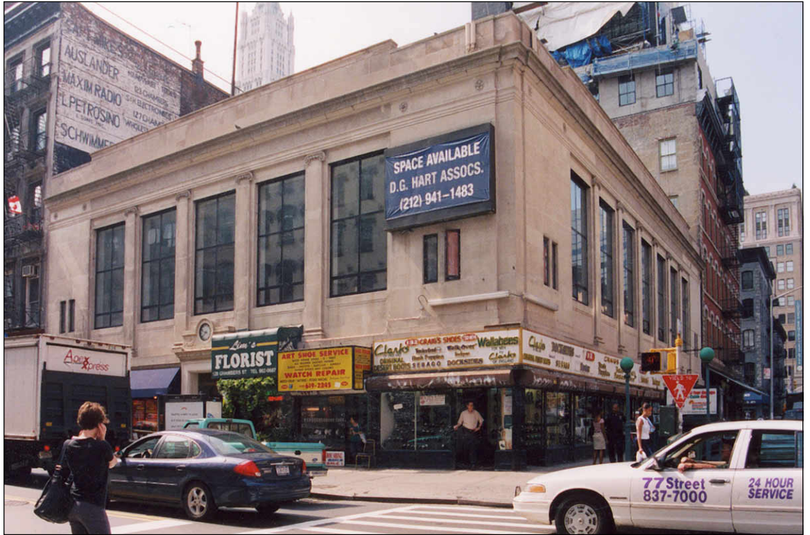
Former Marine Midland Trust Company Building, 128-132 Chambers Street (2003)
