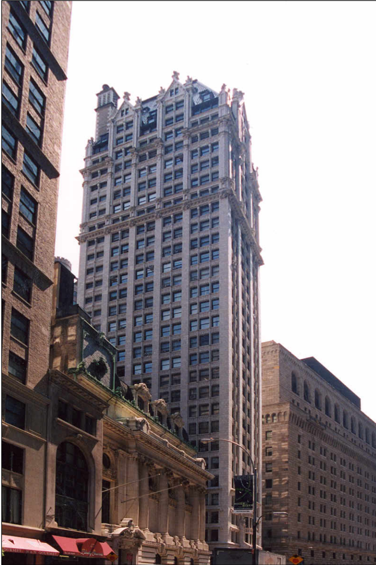
Former Chamber of Commerce of the State of New York (65 Liberty Street) and Liberty Tower (55 Liberty Street) (2003)
