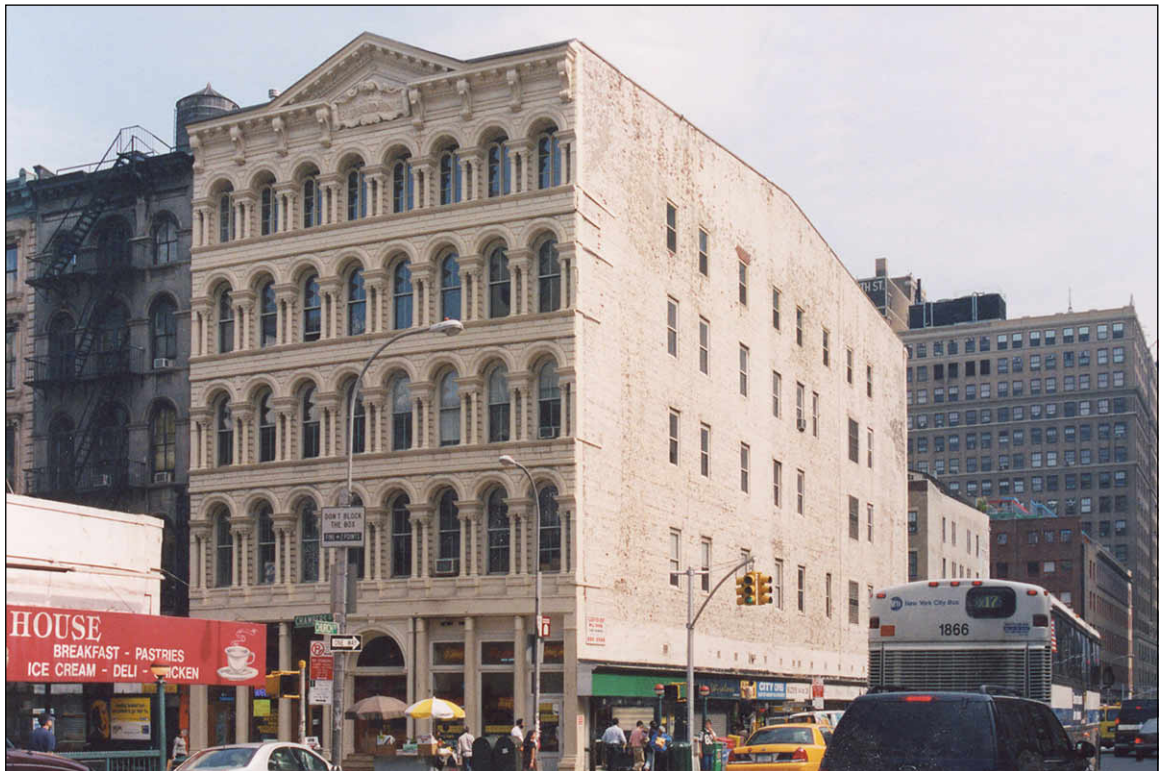
Cary Building, 105-107 Chambers Street (2003)
