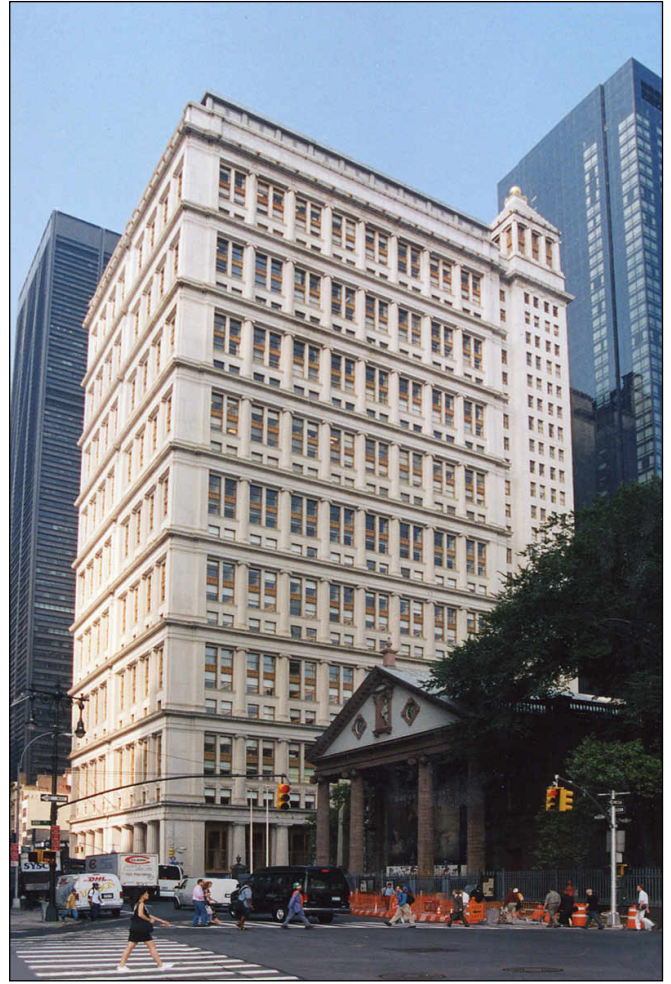
St. Paul's Chapel (Broadway and Fulton) and the former AT&T Company Building (195 Broadway) (2003)
