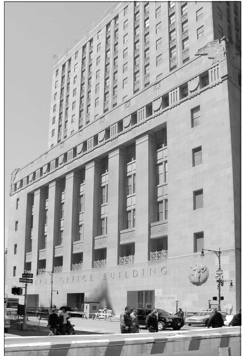
Federal Office Building/U.S. Post Office, 90 Church Street (2003)
